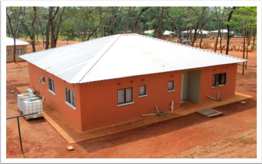
COMPLETED 4-BEDROOM HOUSE 3-JAN-2014
