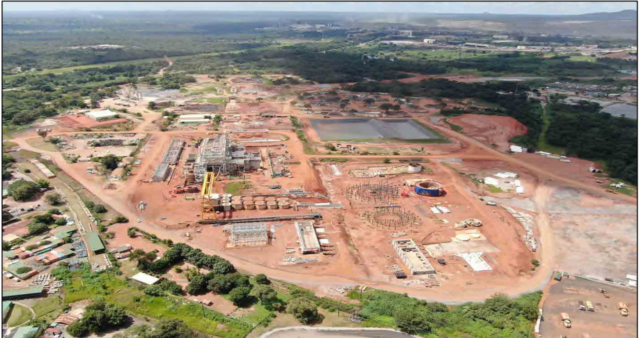
Figure 17-4 Kansanshi S3 plant, partially constructed
