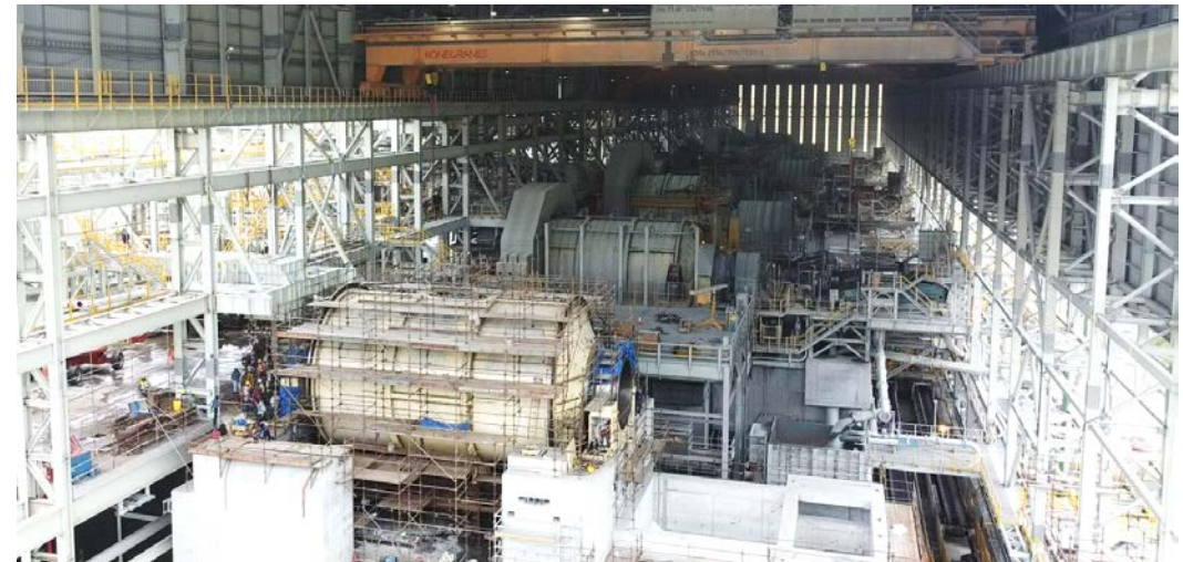
Ball Mill 6 Construction
