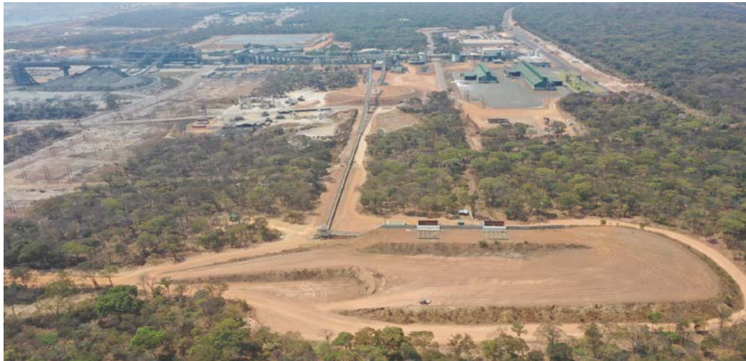
Ore Receiving Area and Crushing
