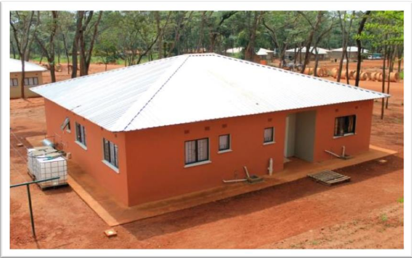
COMPLETED 4-BEDROOM HOUSE 3-JAN-2014
